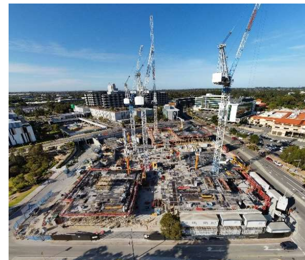
Montserrat's Murdoch Private Hospital in Perth under construction
